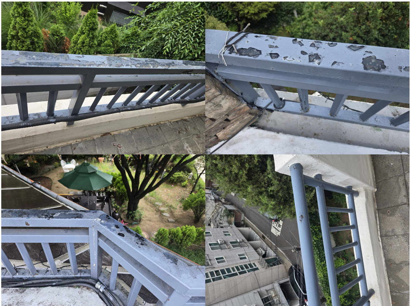
vi. Application of silicon sealant on windows, followed by painting ;included above
